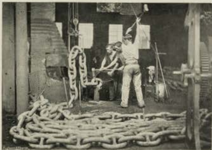
FINISHING A 2½-in. LINK.
