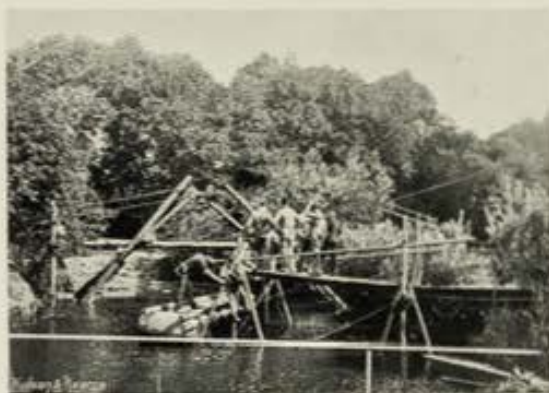
SECURING A TRESTLE.
