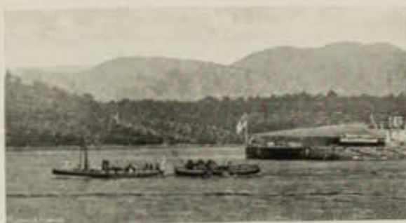
ABOUT TO LAY COUNTER-MINES.
