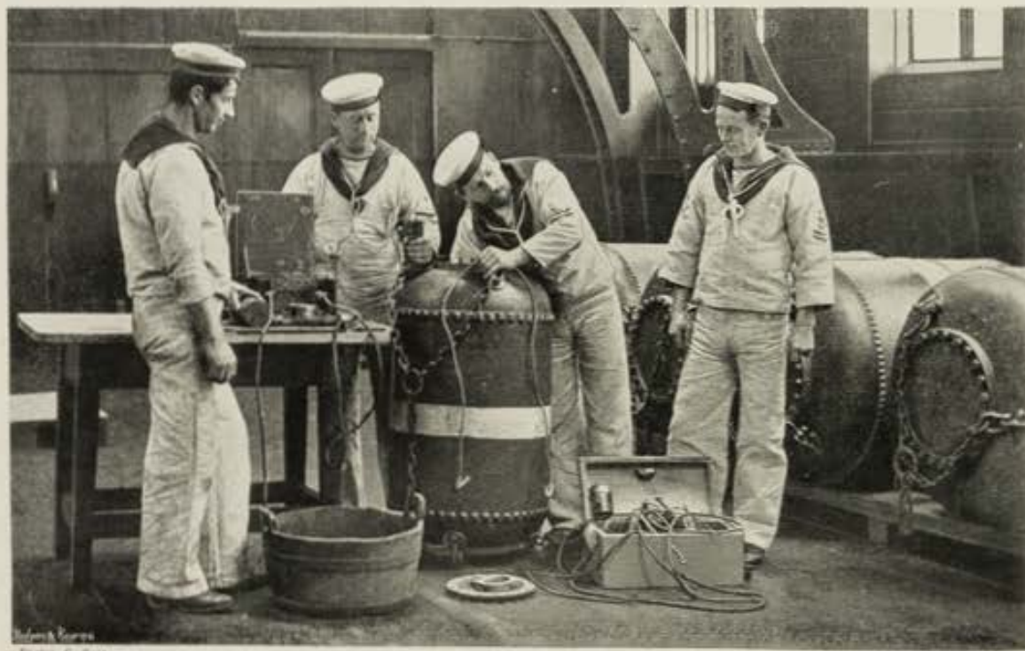
SEAMEN FITTING A MINE CONTAINING 76-LB. OF GUN-COTTON.
