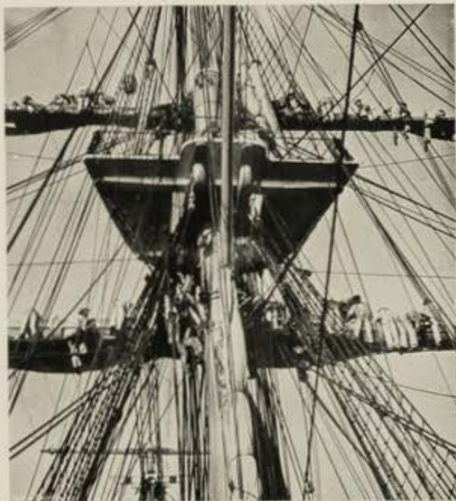
PUTTING ON STEAMING COVERS SEEN FROM AFT.
