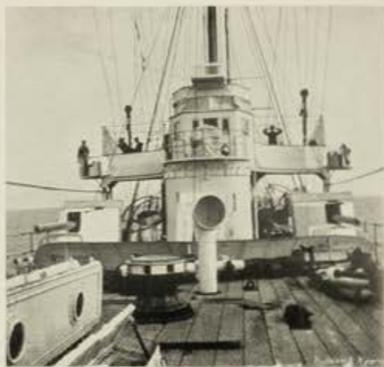
A VIEW OF THE BRIDGE.
