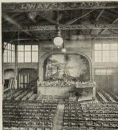
THE LARGE HALL AT PORTSMOUTH
