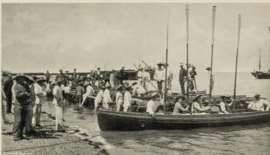
PORTSMOUTH ENGINEER VOLUNTEERS AT RAFT DRILL.
