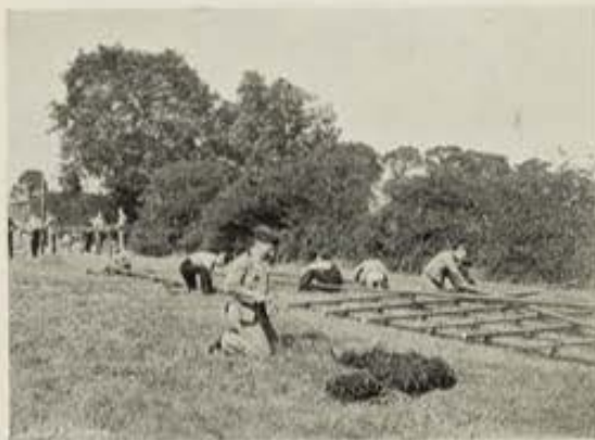
MAKING THE ROOF.
