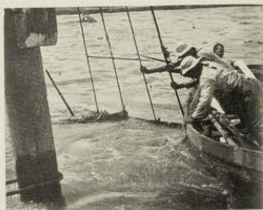
PUTTING DOWN DYNAMITE CHARGES TO REMOVE WRECKS.
