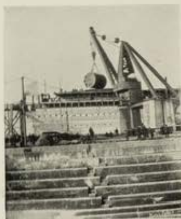
Photo. Kelly. Copyright. LOWERING A BOILER INTO THE "OCEANIC"
