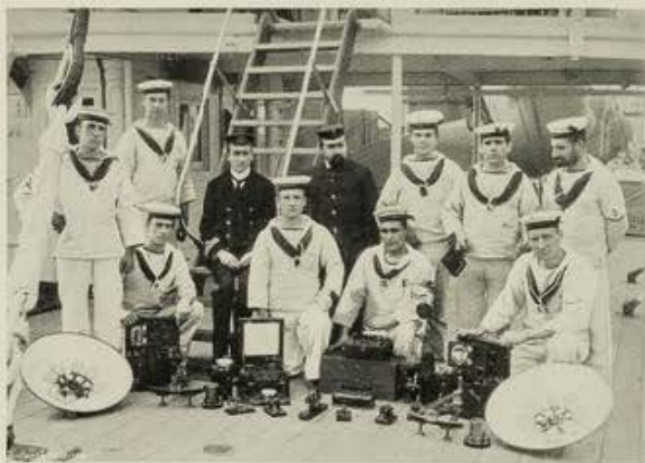
TORPEDOERS AND ELECTRICIANS.
