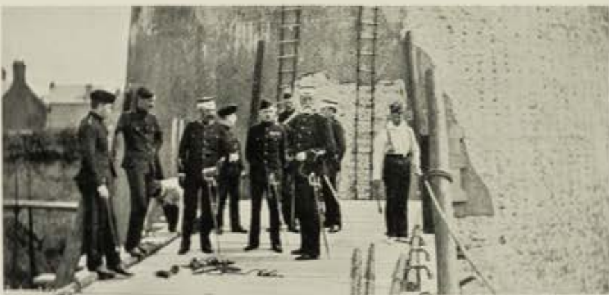
COLONEL WALLER INSPECTS THE WORKS.
