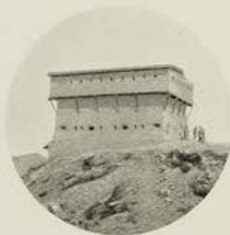
A PICQUET TOWER, CHAKDARA.
