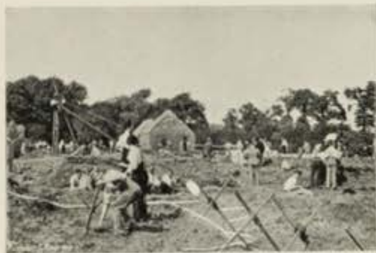
THE TOWER HAMLETS BUSY.
