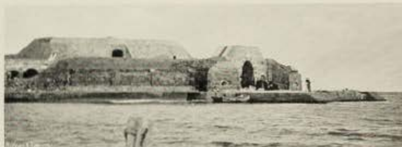
EXTERIOR OF CHANNEL ISLAND FORT.
