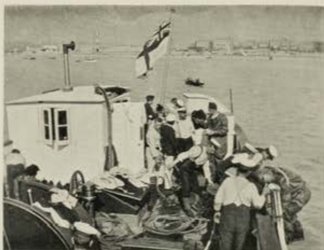
GENERAL VIEW OF OPERATIONS.
